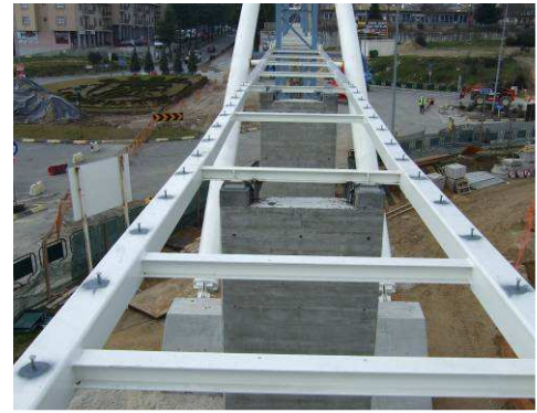
b) Walkway steel girder
