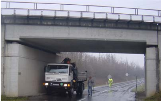
Figure 1 – Bridge 12 (skew): general view
