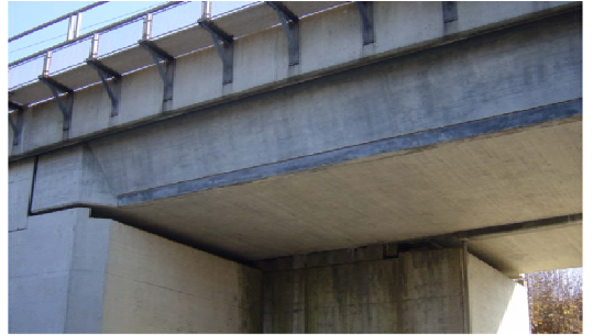
Figure 4 – Bridge 8: view of the abutments area
